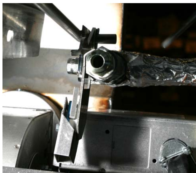
Figure 7: The new micro-switch equipped bracket is shown attached to a drain-flush valve with a left side stem.
