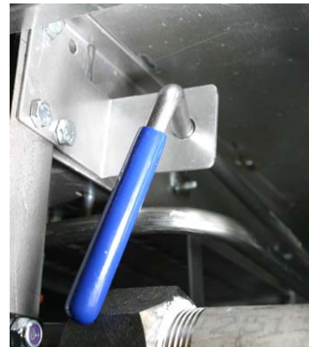
Figure 10: The new bracket for the drain-flush is shown bolted into place. The blue handle is retained from the original drain-flush rod.
