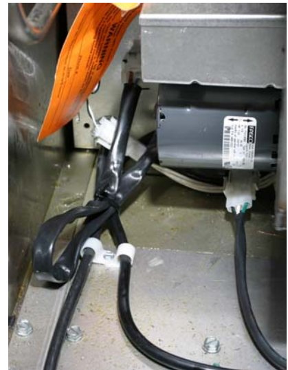
Figure 4: Wires are shown secured with a wire tie on the left side of the fryer (viewed from rear), keeping the harnesses away from the blower housing.
